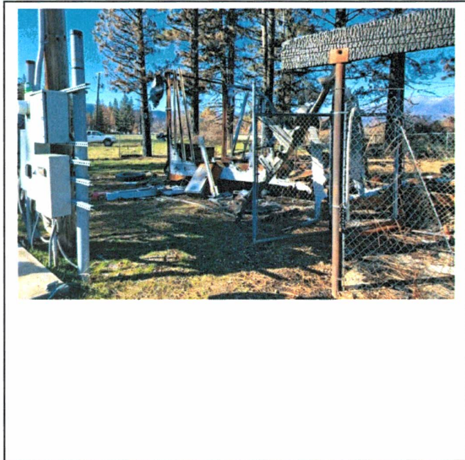
Generator Shed on Right. Trailer remains behind shed.
